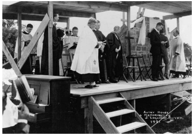
Laying of Autry House cornerstone, June 5, 1921.
