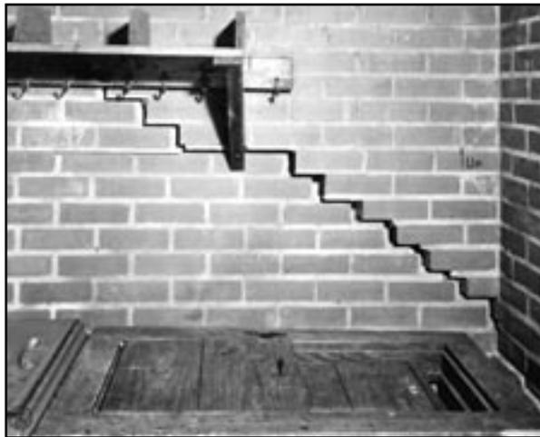
[Old] Field House, The Rice Institute, December 1948. Structural damage to building showing wall damage and movement caused by building sinking and the pulling away of the two story addition on the northeast side of the main building.
