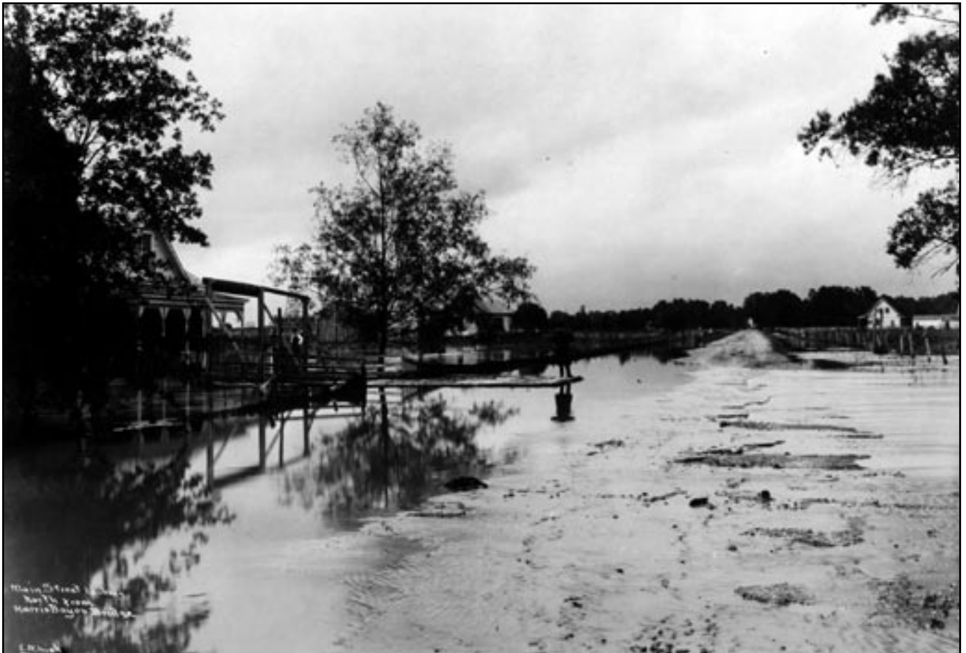
Main Street Looking North, (Rice Campus on left) 1912 Houston, Texas
